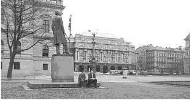
School building viewed from the embankment
